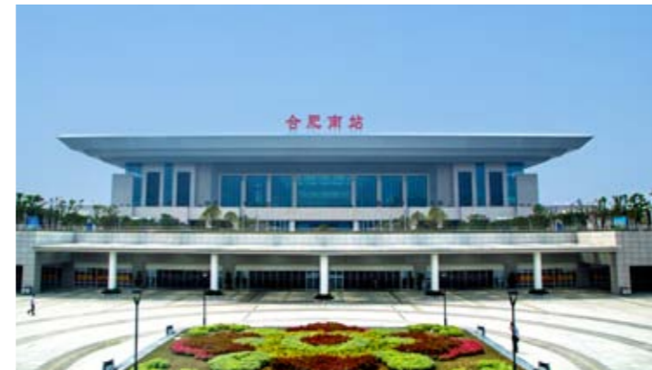
▲ 合肥南站 Hefei South Railway Station
